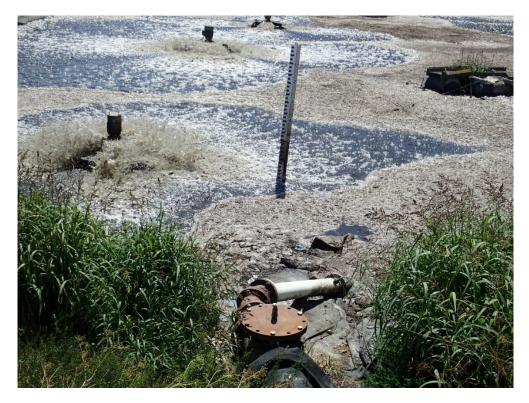
Photo 6 : Pond 1 with level indicator. Note watermark approximately 1.5ft above current level.
