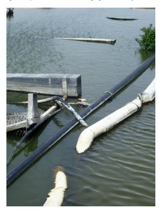
Photo 12 : Baffle in Cell 2C with gap at surface.
