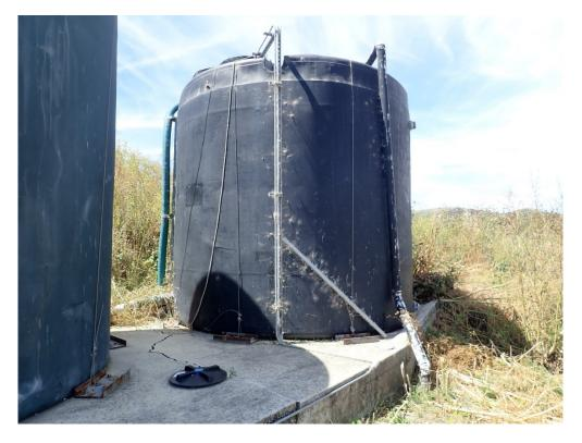
Photo 7: The 10,000 gallon flow equalization tank located between Ponds on the far West side.
