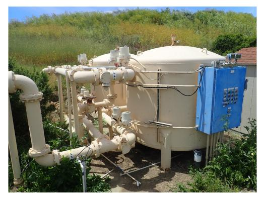
Photo 14 : Pressurized filter system.
