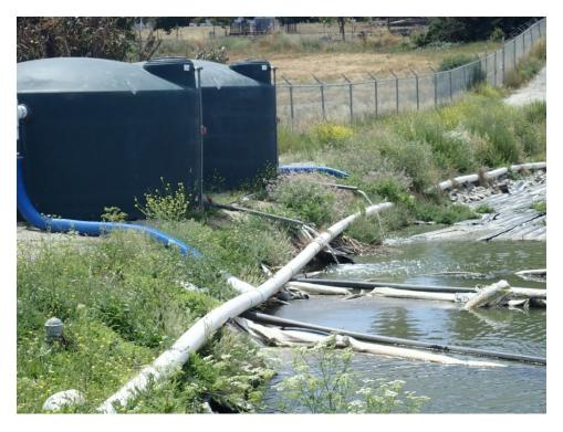
Photo 11 : Two 5,000 gallon equalization tanks discharging into Cell 2C from the East bank of Pond 2.
